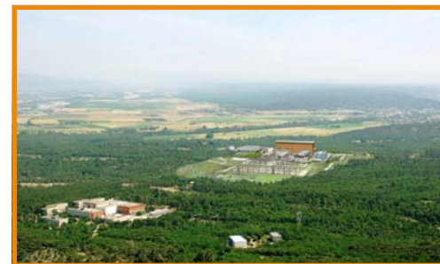
Artist's view of the ITER installation in Cadarache – the Supra Torus installations, the precursor of ITER in operations since 1988, can be seen in the foreground, (© CEA)
